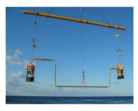
guideline-less techniques. Jumpers or spool pieces are installed after onshore construction and testing to mate to previously installed equipment, based on subsea metrology data.
